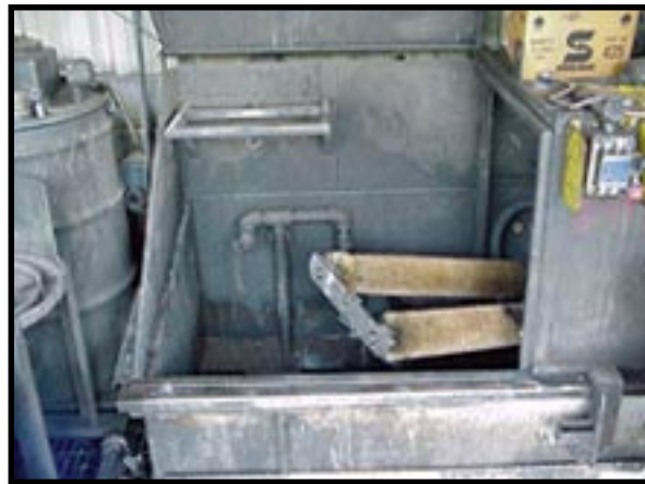
View of interior Drum Washer.
